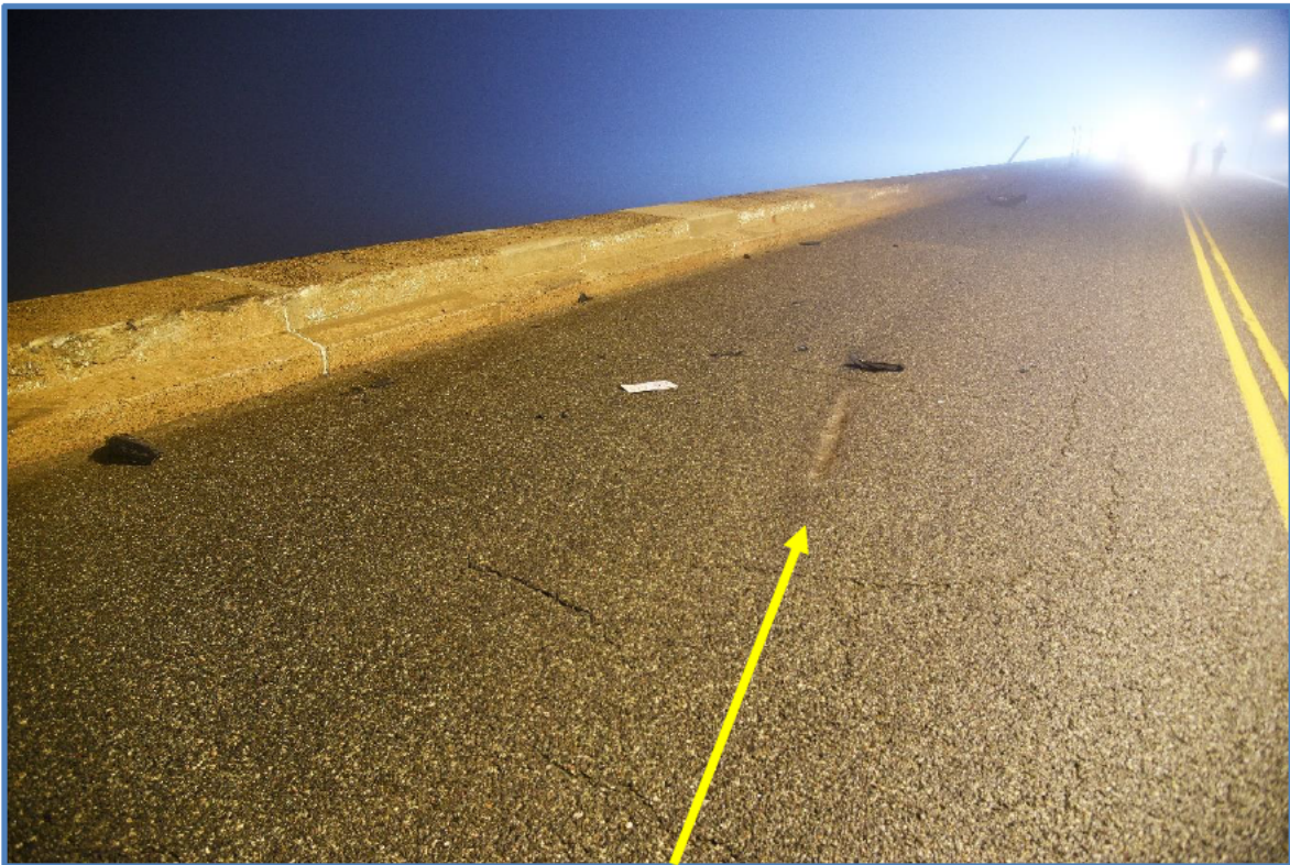
Photo 1 – Tire Gouge/Scrape (Pierce)
